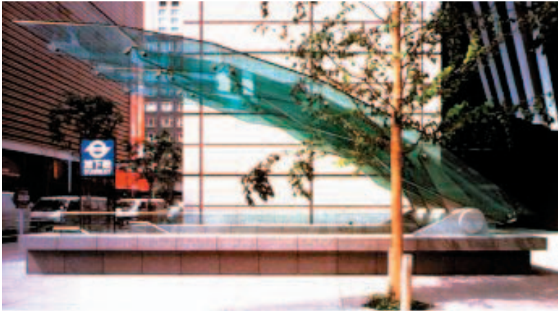
The glass canopy for Yurakucho underground station in Tokyo, Japan.
