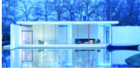
Va-va-voom: One of Firman's supply and fit jobs: Skywood House, Denham, Bucks., location for the Renault Clio advert
